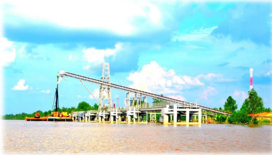
Dolphins & Barge Loading Conveyor
